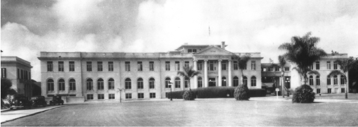
Building 10 (as enlarged, on left), Building 11 (on right), circa 1926. Courtesy of FATCO.
