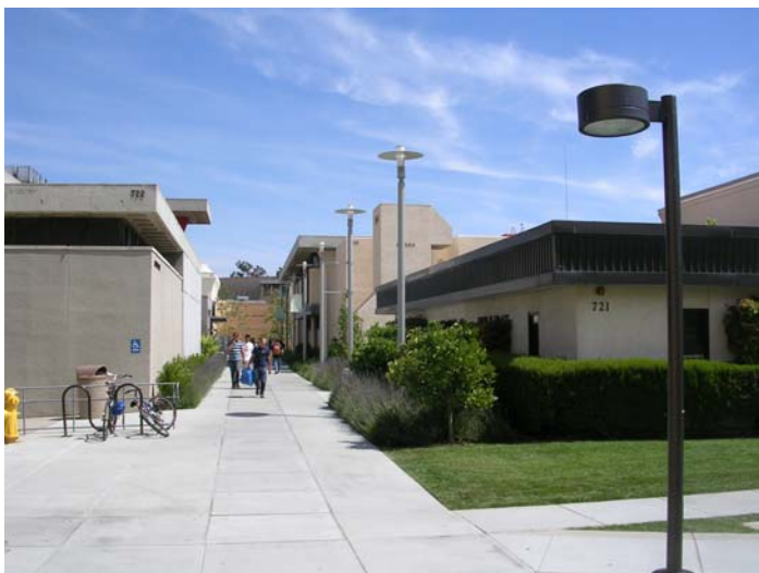
View south along primary pedestrian spine bordered by Arts Studio on the left and Arts Trailer (foreground) and Drama Building (background) on the right.
