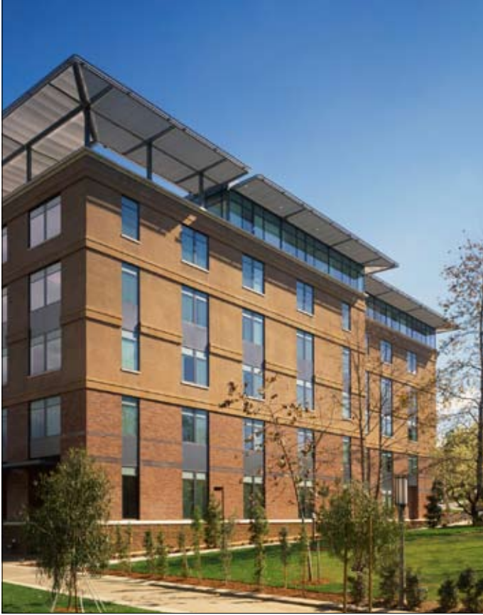
The design of Bren Hall typifies the expression of tripartite building layering, with clearly defined base, mid-section, and roof (A-4) (Photograph by Hedrich Blessing).
