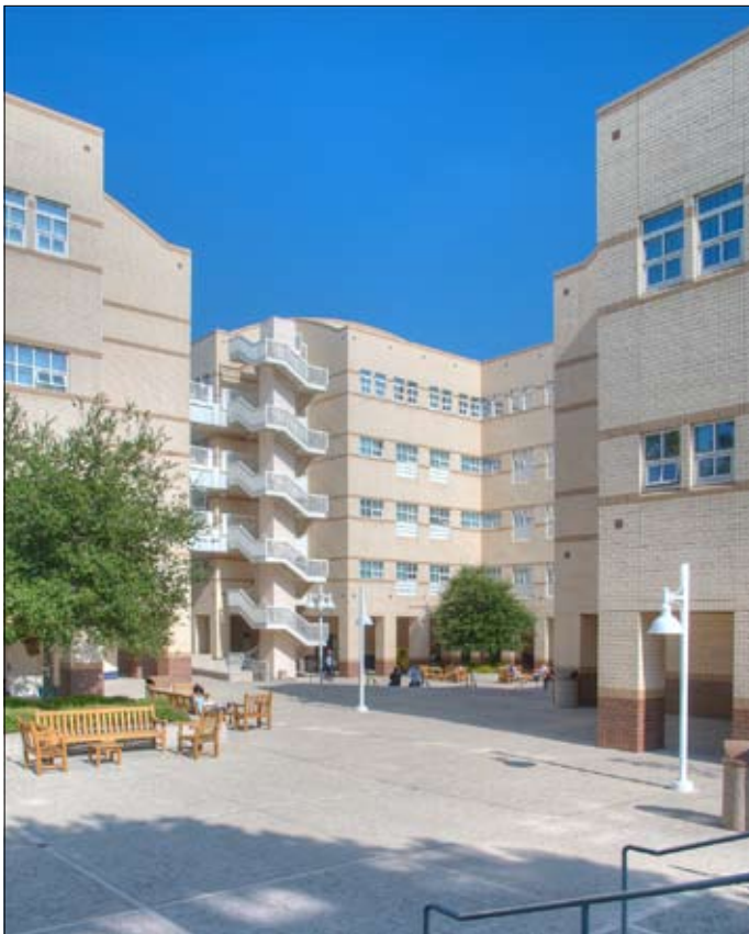
This major public space is defined by the manner in which the Social Science Plaza buildings are sited (SP-14).
