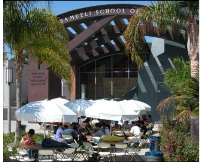
An attractive outdoor space is created at the edge of the Rockwell Engineering Center (SP-17).
