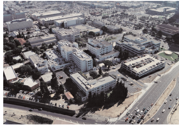
View from north-east
